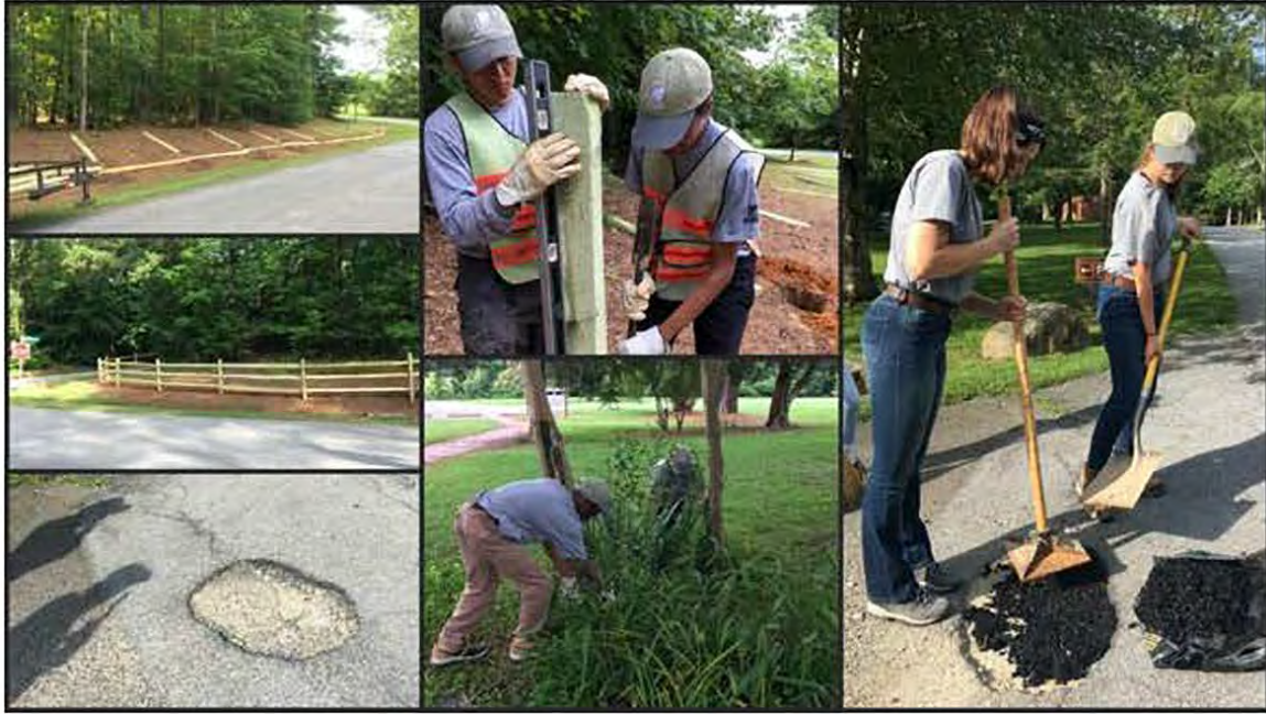
Building fences and restoring gardens at Chippokes Plantation
