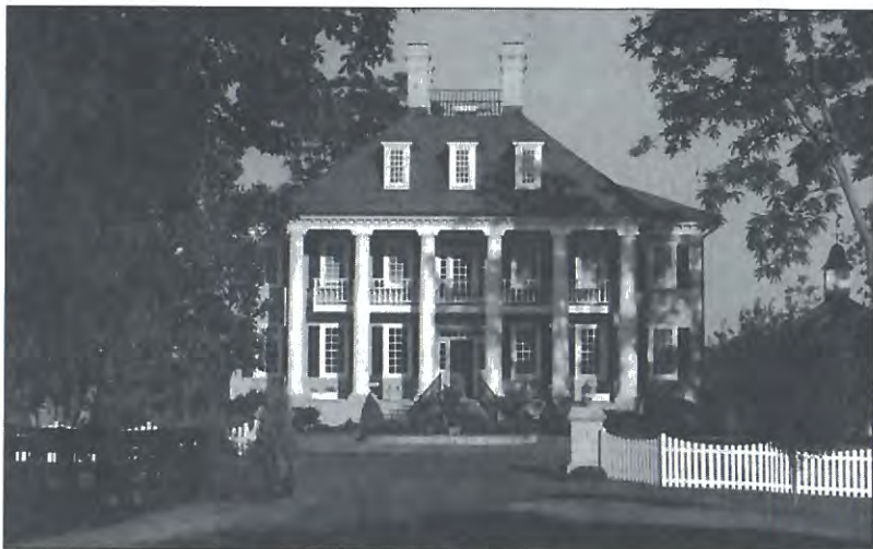
Moriah, a 1988 interpretation of a circa 1833 plantation home from the Savannah River area, is owned by Mr. and Mrs. Steven Rodgers and will be presented to the public for the first time on the Warrenton tour April 21 and 22.
